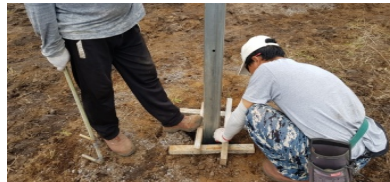
Installing pole structure / fixing with wood supports
