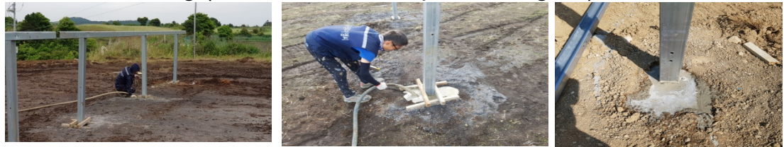
milk-concreting (concrete/water/expansion agent)
