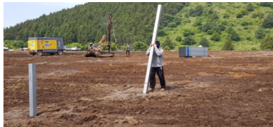
Installing pole structure / fixing with wood supports
