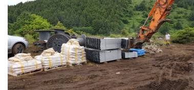
Receiving/loading materials (PosMAC, module, cable, etc..)
